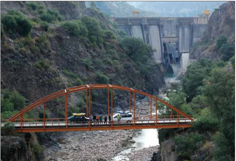
WATERS OF THE MANTARO RIVER FLOW BELOW TABLACHACA DAM DURING THE DRY SEASON.
